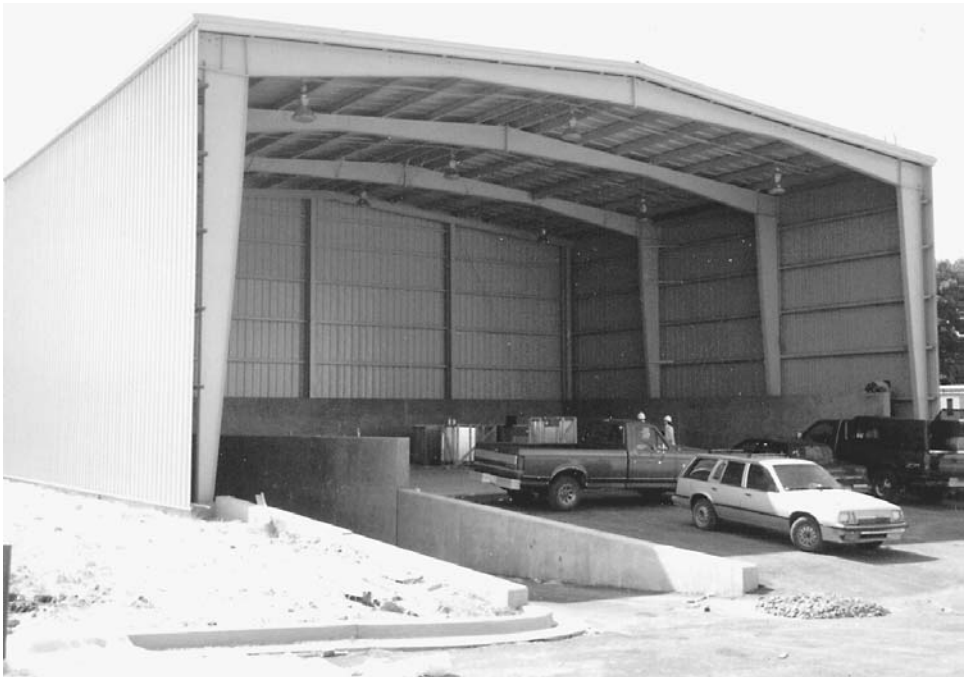
FIGURE 4.9 This open-front industrial facility is ideally suited to single-span rigid-frame construction. ( Photo: Maguire Group Inc. )
